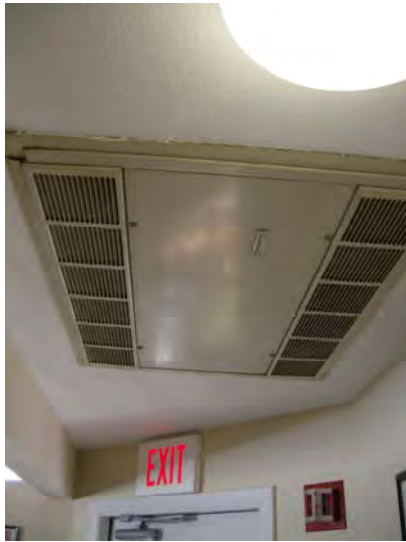
The community room, ceiling mounted electric air handler/heater
