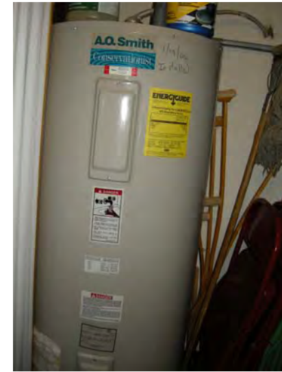
The community room electric water heater
