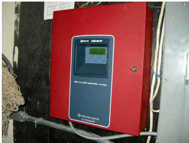
The development's fire alarm control panel
